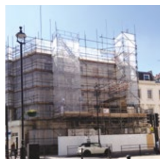
Aud Jebesen Hall during renovations
